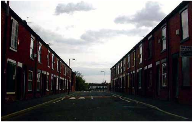
Figure 6-20 Terraced housing in regeneration area
